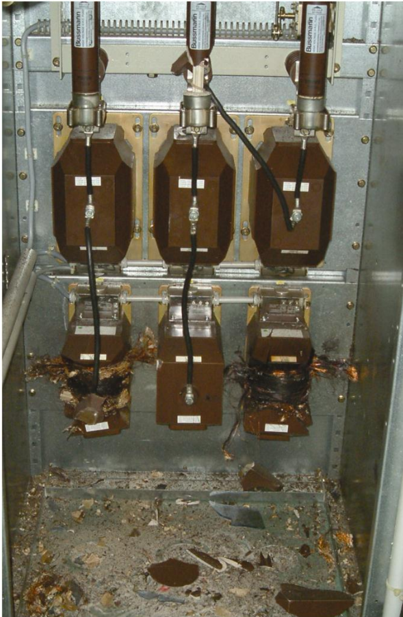
Figure 3: Transformers destroyed by undamped oscillations in the network
