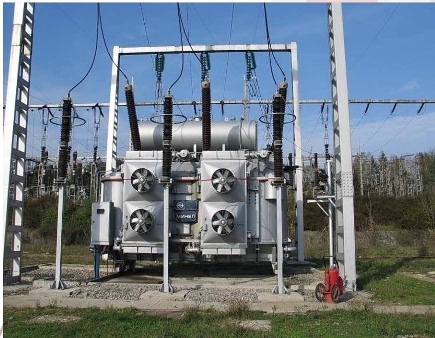
Power transformers rated power 150 MVA, Power Station – Belgrade 8 - Jajinci
