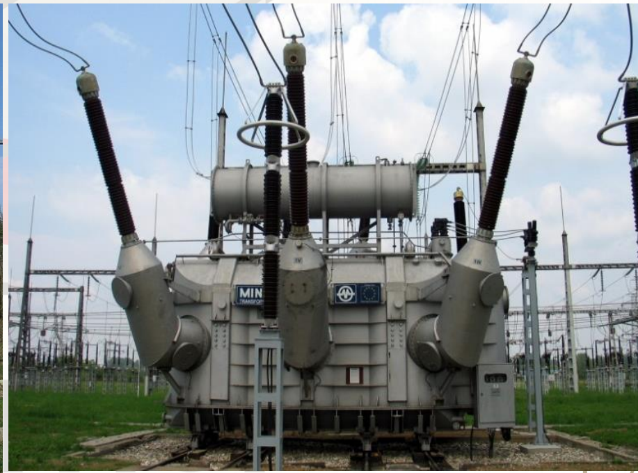
Step-Up transformers, rated power 400MVA Power Plant - KOLUBARA B
