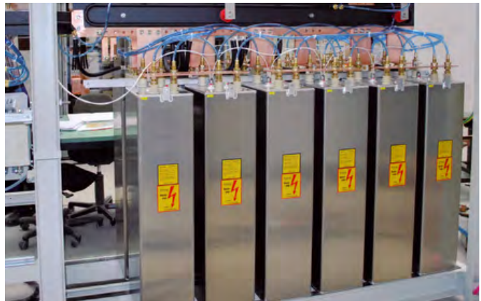
Power electronics with water chiller
