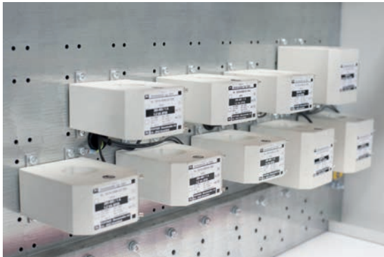
Current transformer installation
