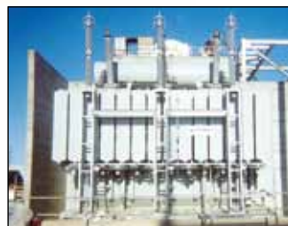
235kV 205MVA Generator Step-up Transformer Sempra Energy in U.S.A.
