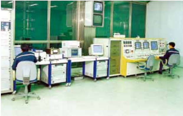
Control Room of Ultra-High Voltage Test Laboratory
