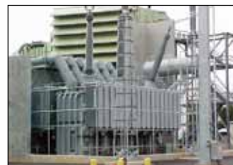
500kV 390MVA Generator Step-up Transformer Tenaska Georgia Power Plant in U.S.A.
