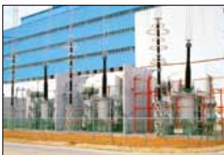
765kV 204MVA Generator Step-up Transformer Dangjin Thermal Power Plant in Korea
