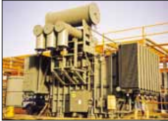
132kV 230MVA Transformer Al-Qaseem Project in Saudi Arabia
