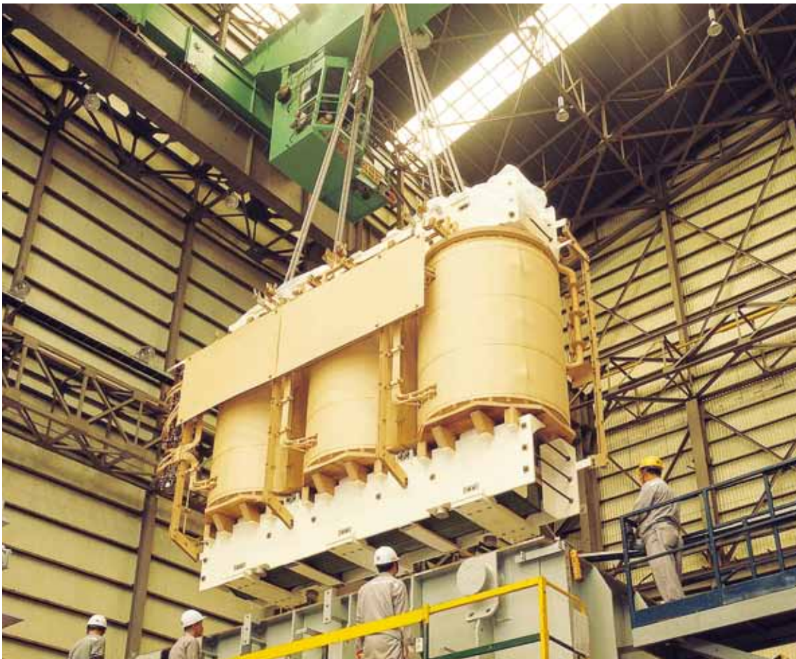
Transformer under In-tanking Process
