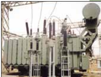
220kV 125MVA Transformer Egyptian Electricity Transmission Company in Egypt
