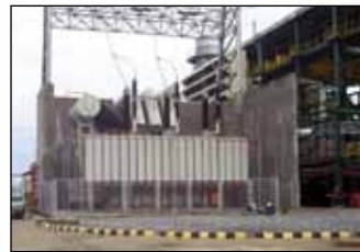
235kV 500MVA Generator Step-up Transformer Bowin Combined Cycle Power Plant in Thailand
