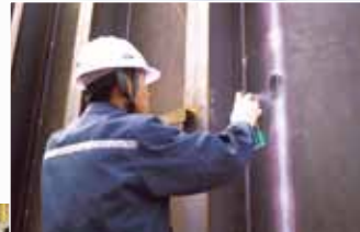
Non-Destructive Test on Transformer Tank
