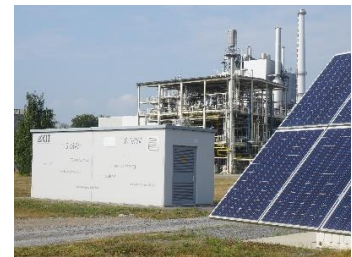
Prototype of a large lithium-ion storage system of the Energy Lab 2.0. (Photo: Battery Technical Center, KIT)
