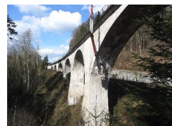
From a mobile platform underneath the Laufenmühle viaduct near Welzheim, radar and ultrasonic measurements were made. (Photo: KIT Innovation HUB)
