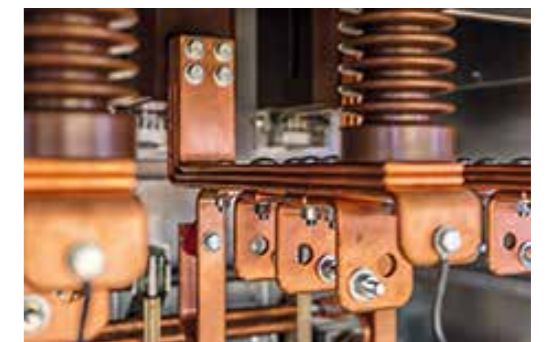
■ Elaborate cable connection.
