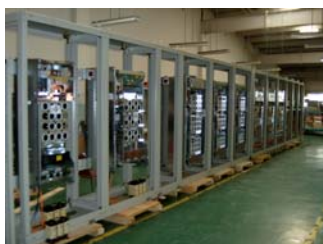
Drive and Inverter engineering and panel building
