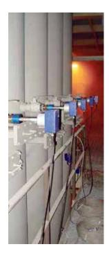
The system is virtually unaffected by pressure and temperature and provides a typical accuracy within +/- 5 % in pneumatic conveying systems (with even deviation of the product). The sensor can be use to monitor and control the solid flow in vertical pipes and pneumatic feed lines. For pipe diameters above 250mm it could be necessary to install 2 or 3 sensors for a better coverage of the particle flow profile.
