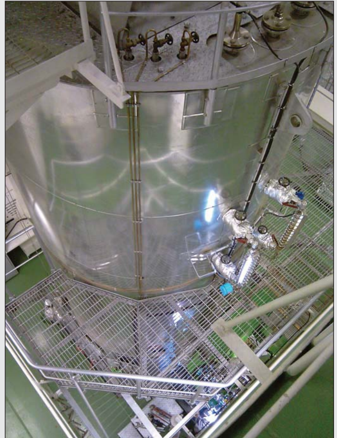
Marine Auxiliary Boiler
