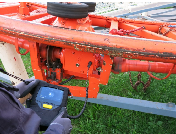
The new VIBSCANNER® 2 can record all the measurement data in just a few seconds. In this regard, a total of 76 measurement locations need to be recorded. These measurement locations are located up to 54 m above the ground.
