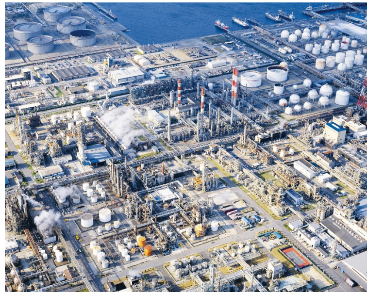
The failure of a single system can entail serious consequences.
