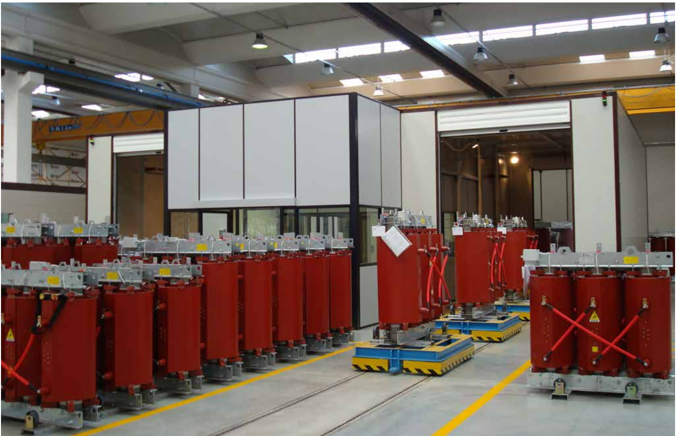
Testing bay for cast resin transformers
