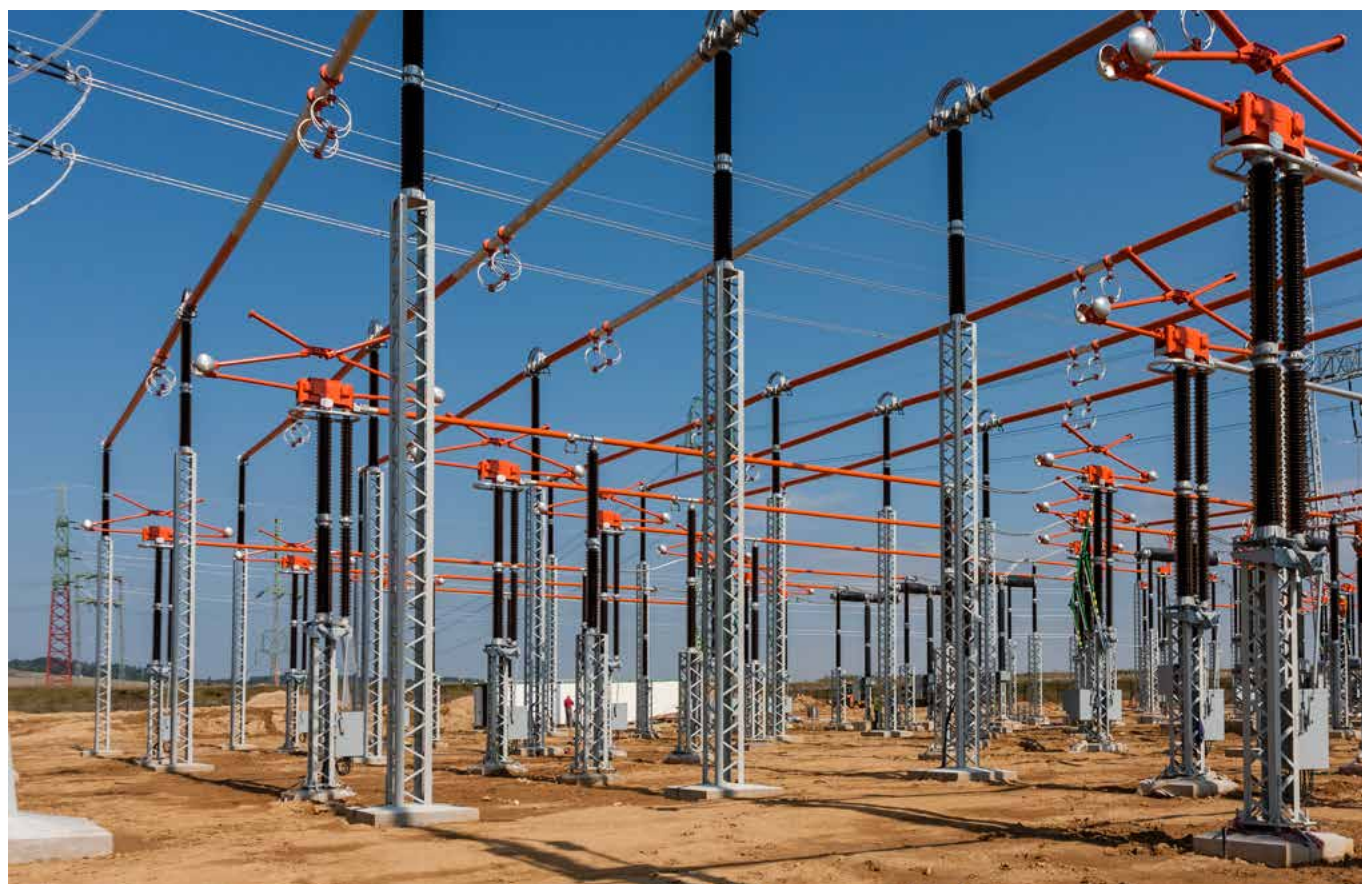
Pantograph disconnectors installed in a 420kV substation
