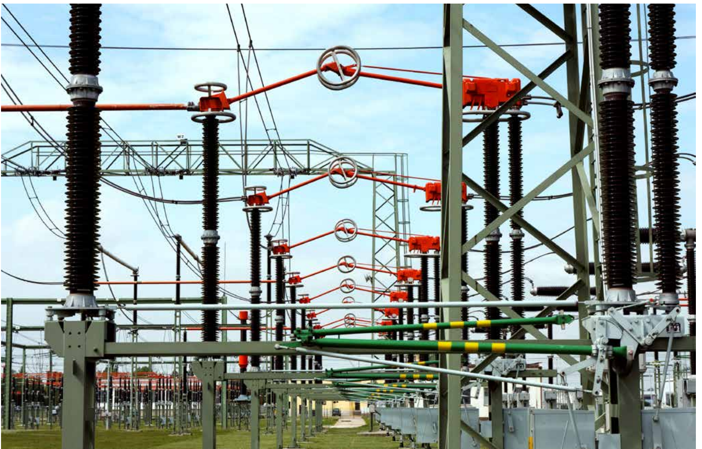
Vertical disconnectors 420kV with earthing switch
