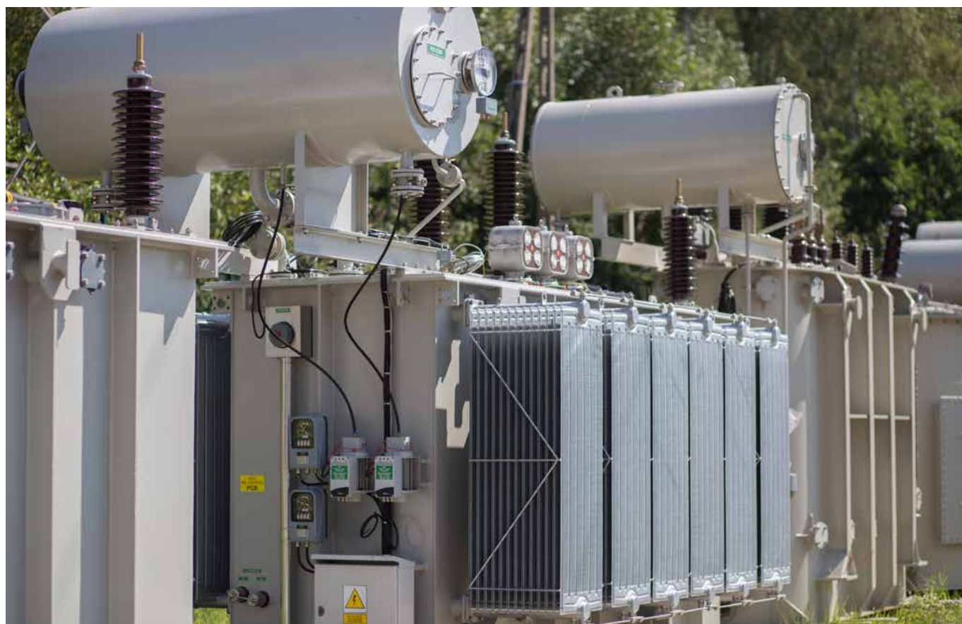
Power transformers waiting for transport
