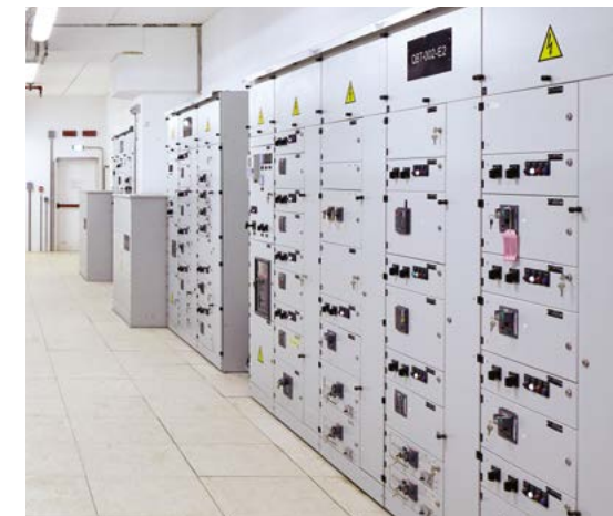
Low voltage main distribution switchgear and motor control center
