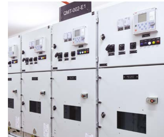
12 24 kV Air insulated medium voltage switchgear for primary distribution
