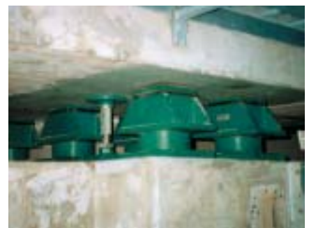
TFD plate spring beneath a foundation
