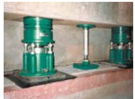
TFD plate spring beneath a foundation with support element
