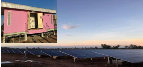
50MW PV station in Thailand
