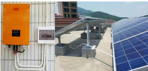
Rooftop PV system in Yangjiang
