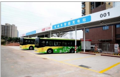
Electric Vehicle Charging Station in Dongguan
