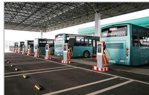
Electric Vehicle Charging Station
