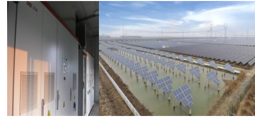
50MW PV station in Jiangsu
