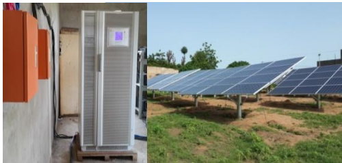
PV station in Mali
