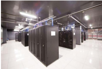
Guangdong CMCC data center
