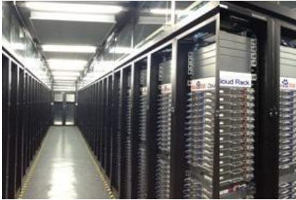
Baidu IDC data center
