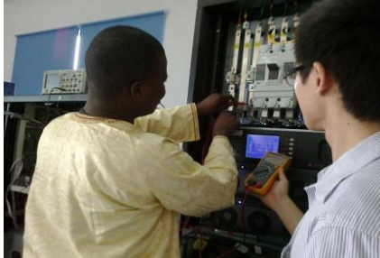
200KVA modular UPS in Mali
