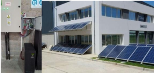
Rooftop PV system in Argentina
