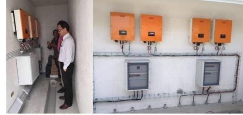
On-grid inverter in Guatemala
