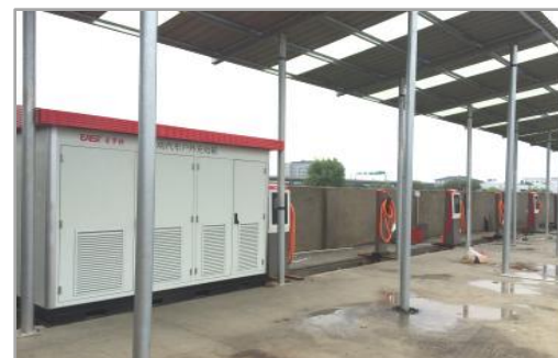
Electric Vehicle Charging Station in Changzhou
