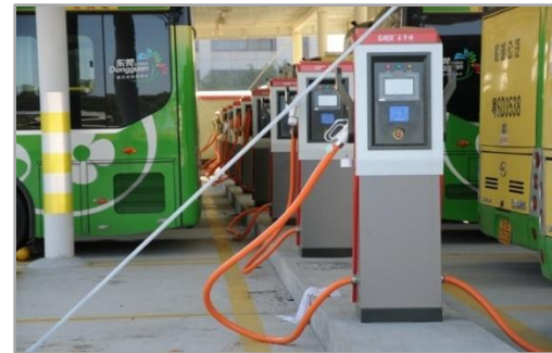
Electric Vehicle Charging Station in Dongguan
