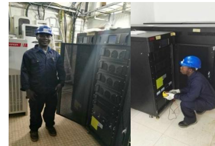
20KVA, 60KVA, 100K VA modular UPS in Africa telecom
