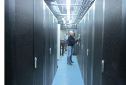
200KVA modular UPS in Jordan telecom
