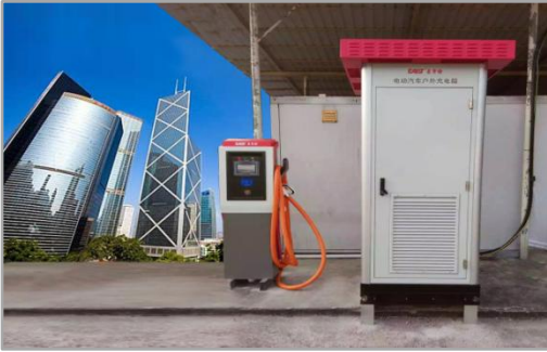
Electric Vehicle Charging Station in Hong Kong
