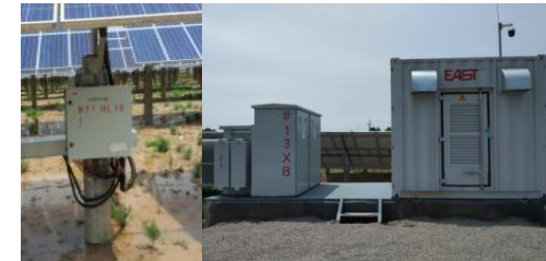
PV station in Shandong
