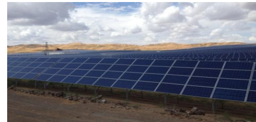
500MW PV station in Ningxia
