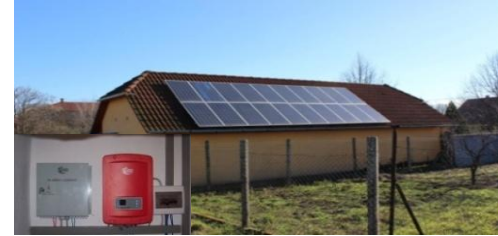
Rooftop PV system in India
