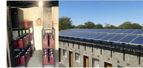
Rooftop PV system in Africa
