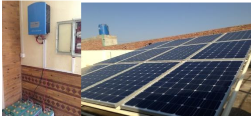
Rooftop PV system in Pakistan
