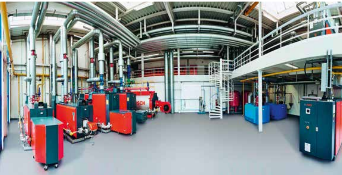
Central power plant at Bosch Thermotechnik GmbH in Lollar (picture by Bosch KWK Systeme GmbH)
