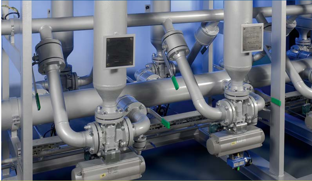
Detail of a Modular Filter Unit Type RSFA 27
