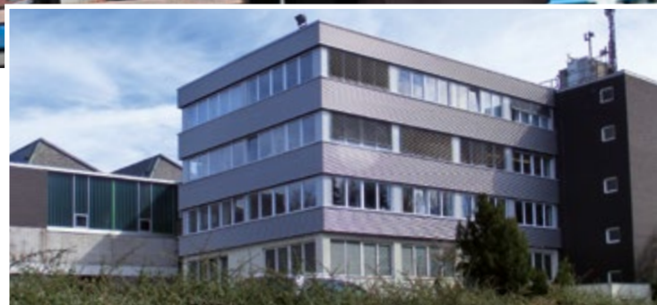
KÖBO industrial park Wuppertal
