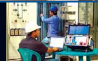
Testing and commissioning in progress at Rabigh power station
