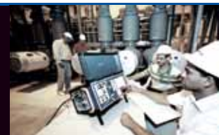
GIS testing in progress at the 380kV PP8 substation at Riyadh
