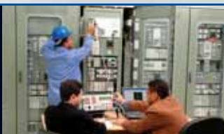
Engineers performing SOE, Fault Recorders Test
