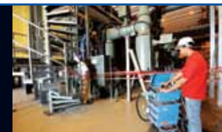
Primary current injection test in progress at PP8 project in Riyadh
