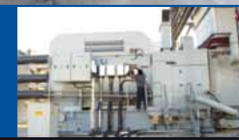
Engineer at work for Generator Testing
