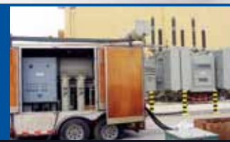
Mobile Oil Treatment Machine at work at Ras Al-Zour substation
