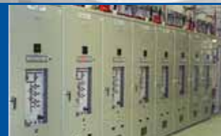
Complete Testing at 380kV Substation at Rabigh
