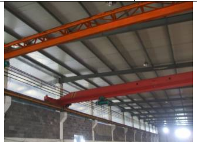
Photo 8 Travelling crane(Max. 3t)
