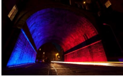
The Regent Bridge Edinburgh, UK
