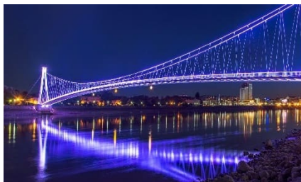
Osijek Bridge Osijek, Croatia
