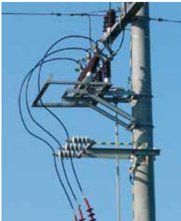
protection of MV cable – outlet of overhead line
