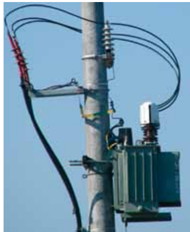
protection of simple transformer station 15/0,4kV
