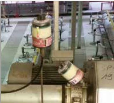
The running time per filling is adjusted directly on the device. The remaining filling cycles are shown by LEDs.
