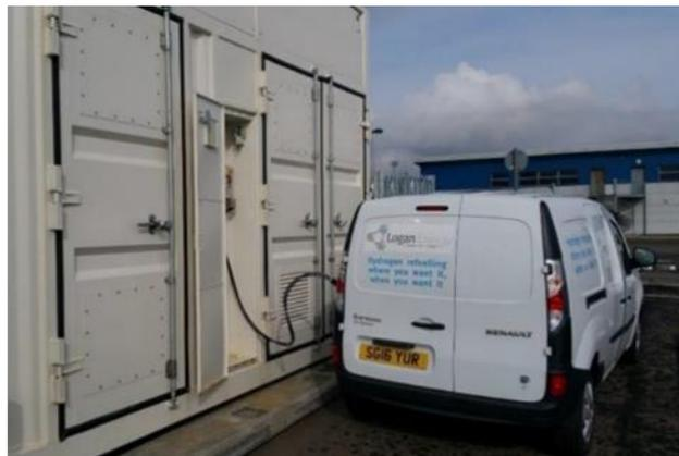
All pipework, valve and safety systems were designed, selected and installed by Logan Energy. Pressure testing of the equipment under the Pressure Equipment Directive requirements (PED directive 2014/68/EU) was also undertaken by Logan Energy and the whole hydrogen system was CE certified.
