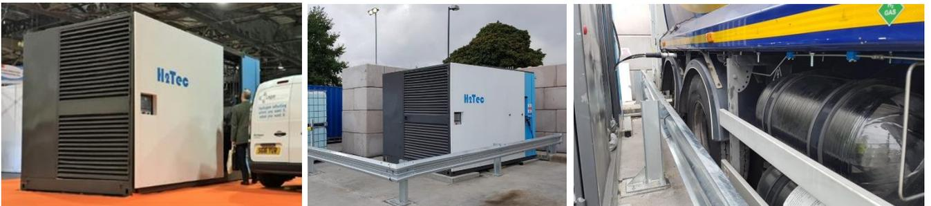
Alongside the containerised hydrogen refuelling station, we have installed a containerised alkaline electrolyser, which will generate the hydrogen dispensed by the refueller. This electrolyser is supplied by de-ionised water and is connected to the local power grid.
