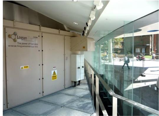
The fuel cell forms part of an integrated tri-generation system providing electrical energy, heat and cooling to the Palestra building. It is the largest capacity fuel cell operating in London.
