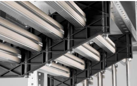
INCLINED BUSBAR HOLDERS
