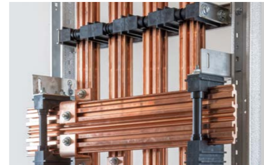
BACK COPPER BUSBAR HOLDERS
