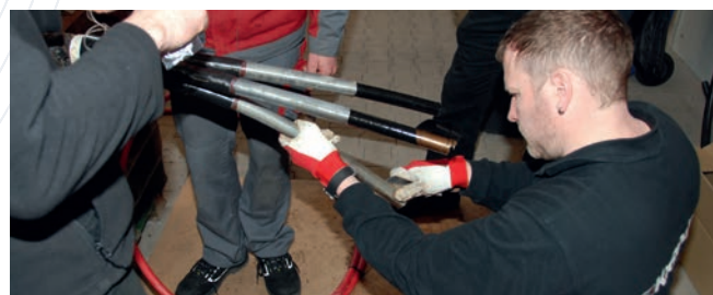
Course in joint installation
