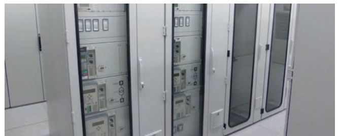
1990 | Introduction of digital protection equipment technology
