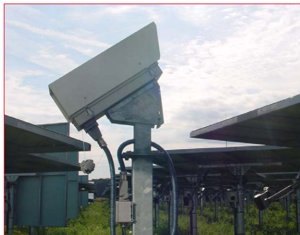
Protected acquisition unit
