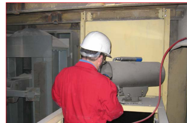
Professional system installation
