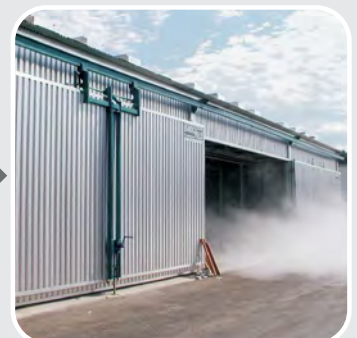
Complete timber drying plant.
