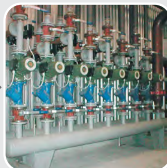
Hydraulic plant for heating fluid feeding.
