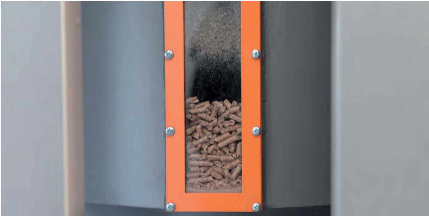
Sichtfenster der Brennstoffschleuse am Gasreaktor. Window of fuel lock near by the gas reactor.
