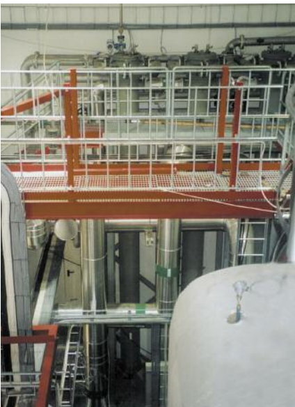
4 MW water/water heat exchanger for district heating with removable covers
