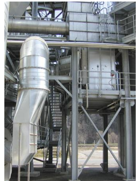
water/air heat exchanger for preheating combustion air; 71,00 m 3 /h; 1.56 MW
