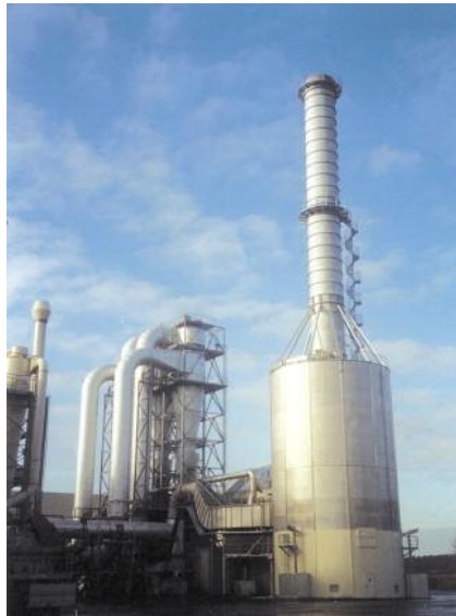
DUAL WESP in stainless steel 2 x 266,000 Am 3 /h; 60 m stack height
