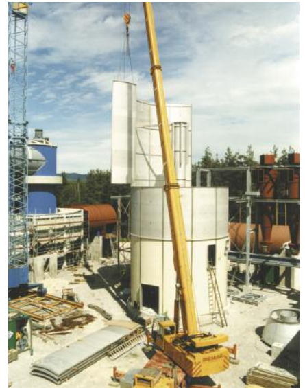
Panel construction in stainless steel with pre-assembled bearing edges on the central support
