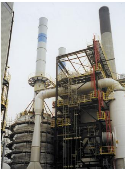
Exhausts of liquid waste incineration with 2 DUAL WESP; 4 x 118,000 Am 3 /h
