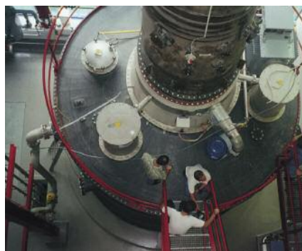
Waste incineration with WESP after Dry EP and Scrubber; 2 x 90,000 Am 3 /h
