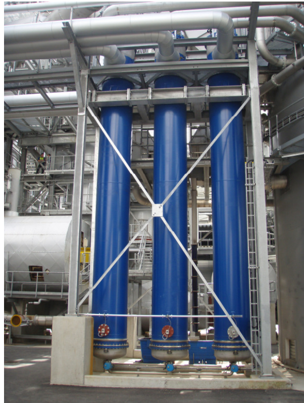
Water/Water Heat Exchanger 3 x 4 MW • 72 °C outlet for district heating
