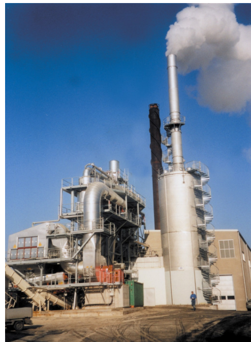
Pellet drier with wet absorber, wet electrostatic precipitator and water/water heat recovery system
