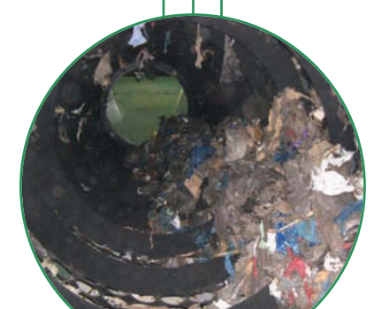
Drum Screen interior view
