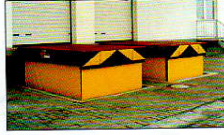
Hydraulikaggregat extern Hydraulic unit external
