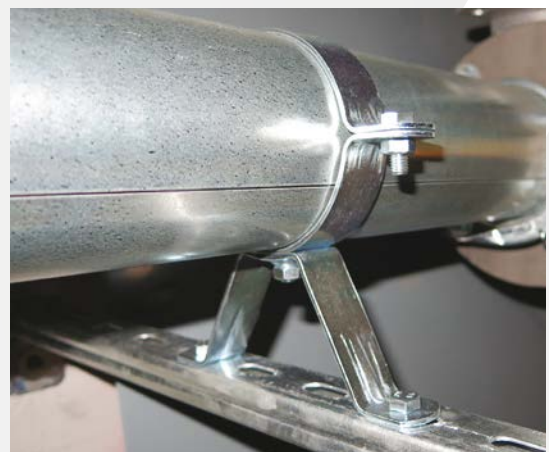
Straight Duct mounted with Split Strap and Legs for Split Strap.
