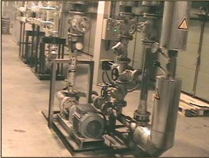
Automatic temperature control system for thermal oil with circulating pump and modulating 3 way valve for each control zone.
