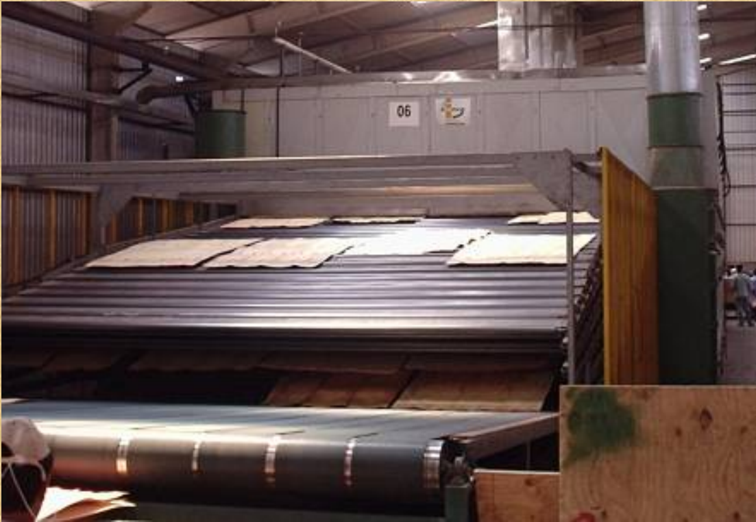
Dryer out feed with unloader conveyor
