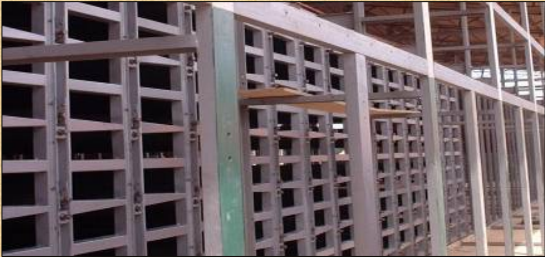
Heavy frame of laminated steel beams treated and painted with special and resistant paint.
