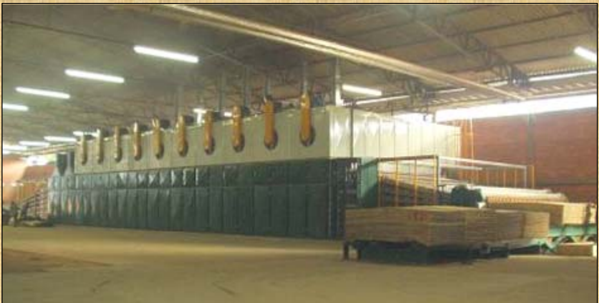
Fan system with external motor, shaft, pulleys and "V" belts allowing less electrical energy consumption and easier maintenance.
