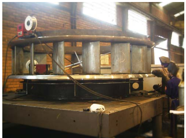
- Welding operation – Hydroelectric power plant distribution body
