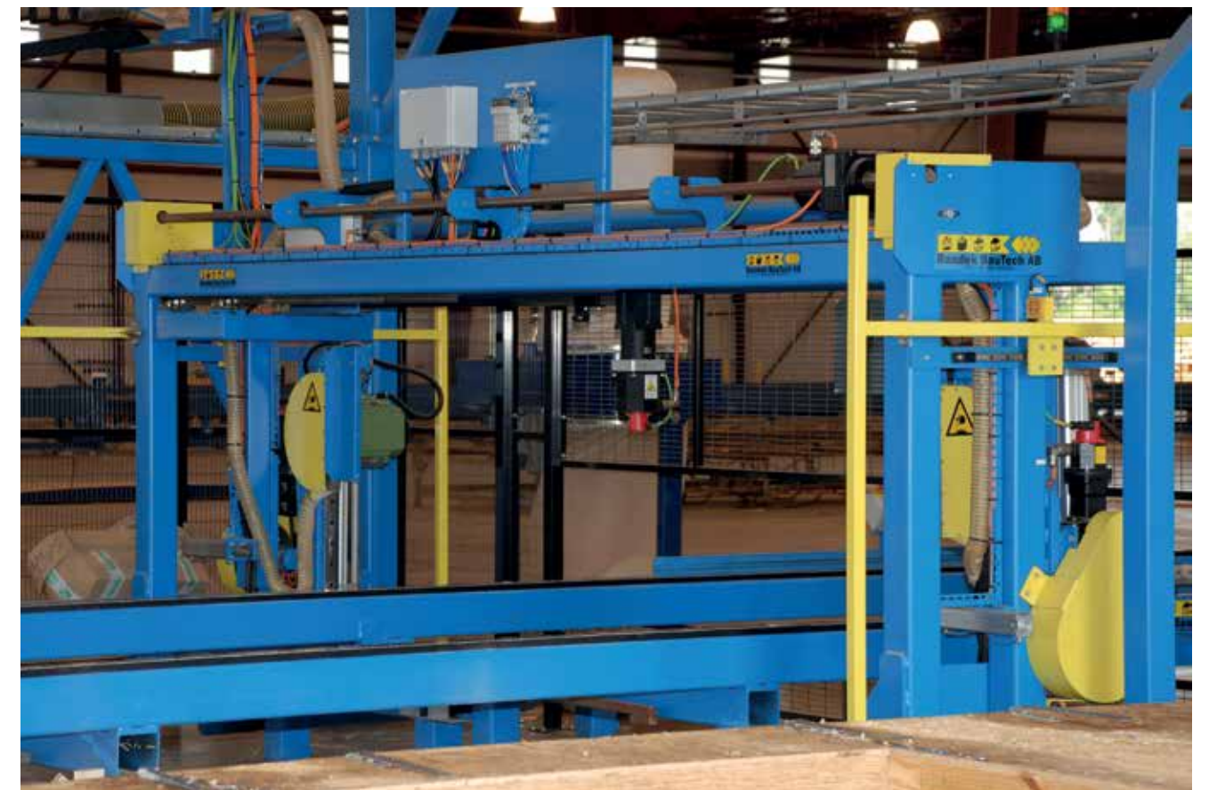
Wall Saw station
