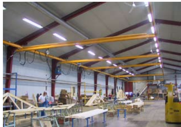
Press line in light overhead crane
