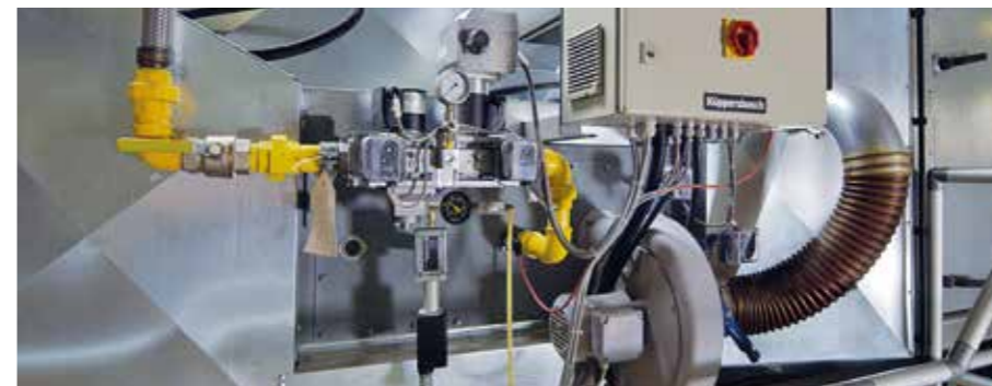
Modern and energy-efficient drying systems
