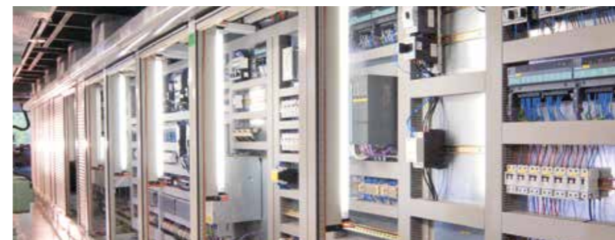
Modernisation of machine control
