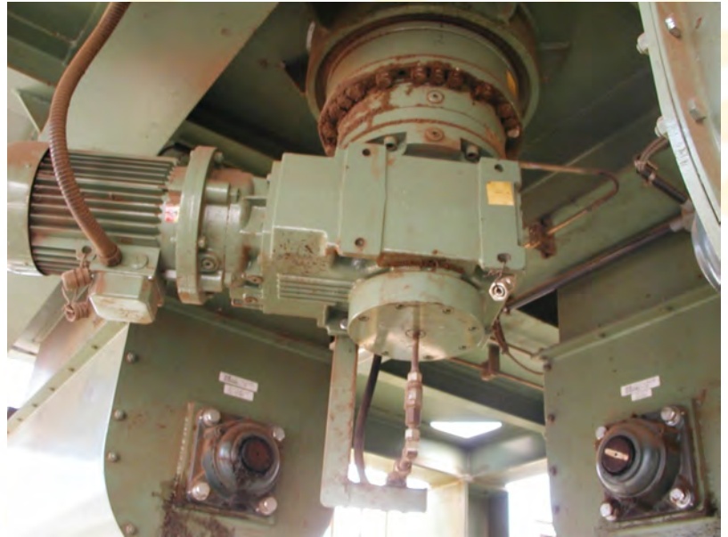
Hydraulic Rotor System with Planetary gear motor with gear box and screw in star arrangement
