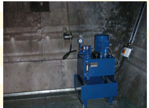
Hydraulic power pack for activation of rotor arms
