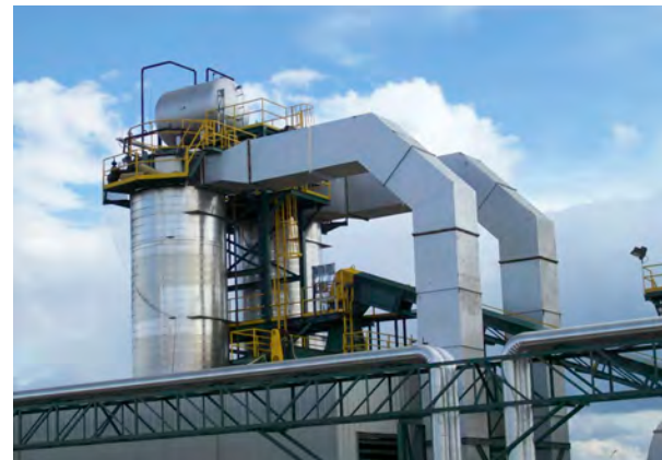
FIG 6.4 Biomass Fired Thermal Oil System
