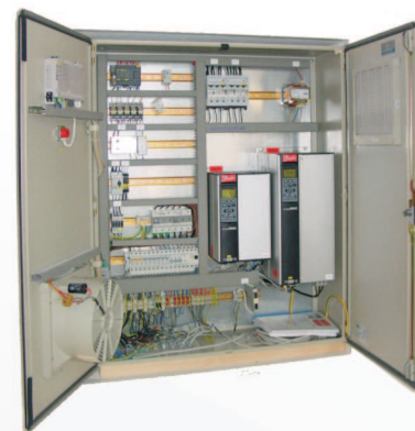
switch board exhaust unit
