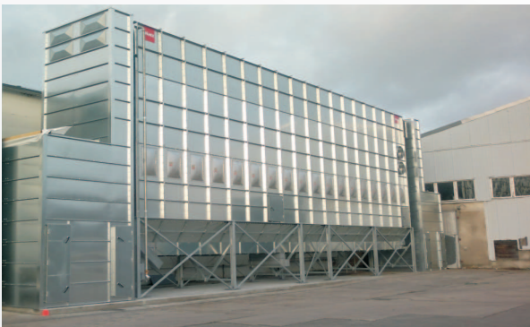
line filter with reverse-air cleaning
