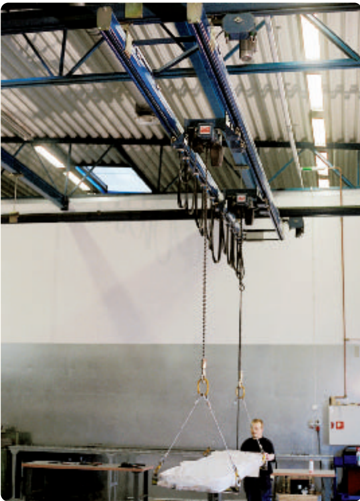
The steel industry uses Lyftman twin girder crane with motorized trolleys.
