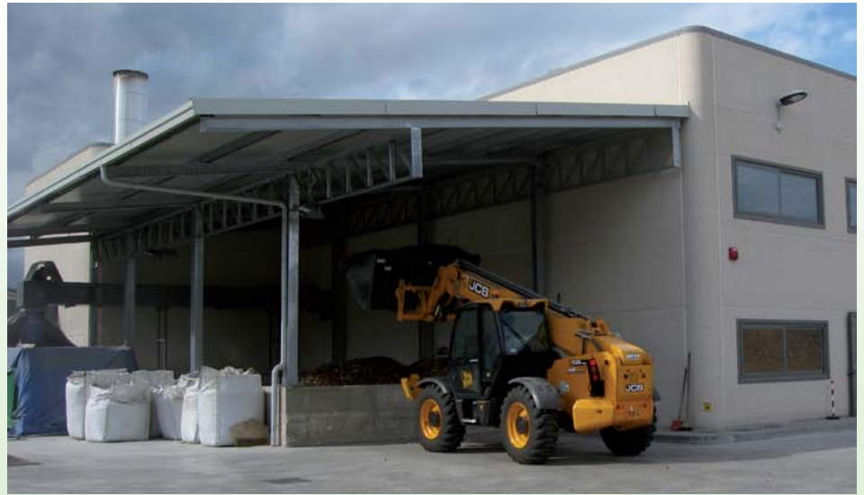
Up: biomass discharged in silo. Down: biomass stocking on the external square
