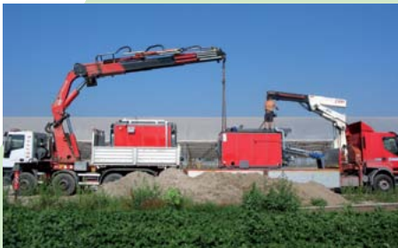
Stages of boiler installation
