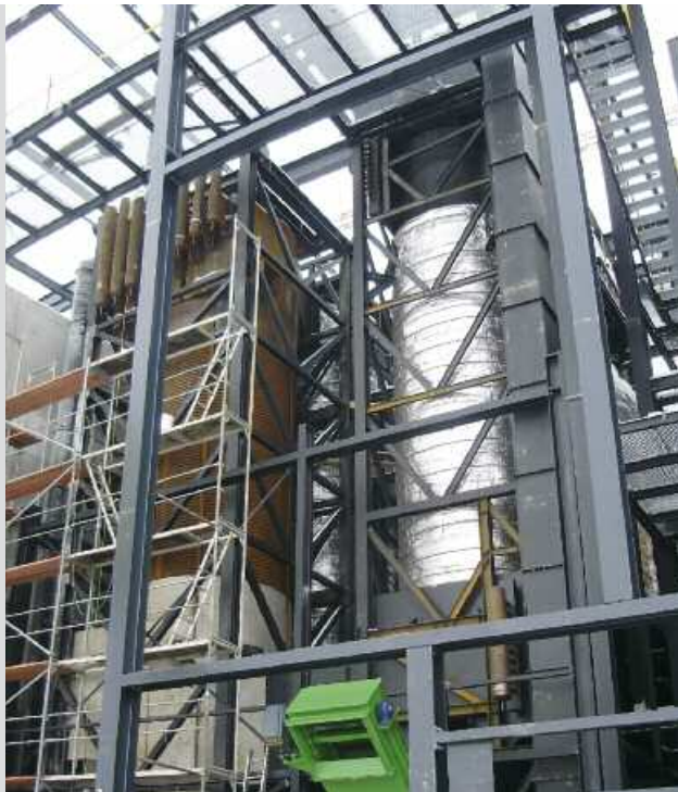
picture of installation
