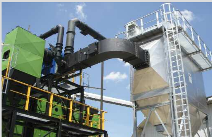
picture of installation
