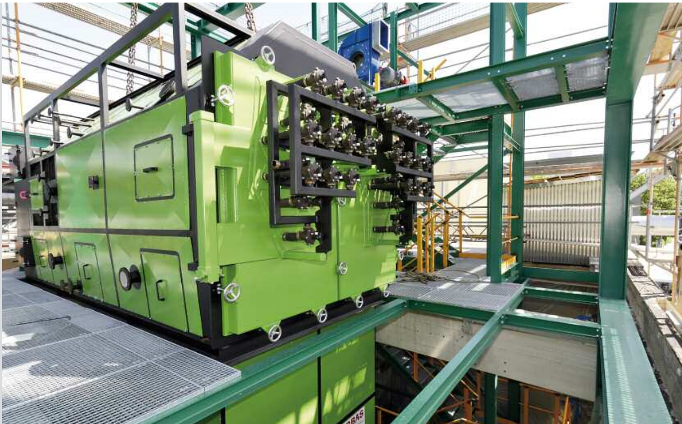
picture of installation
