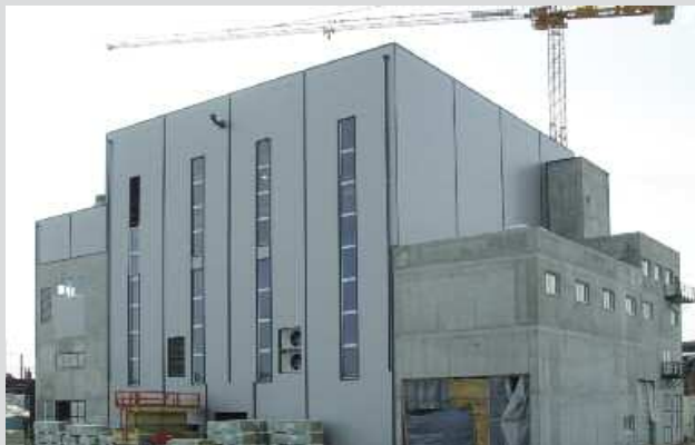
picture of installation
