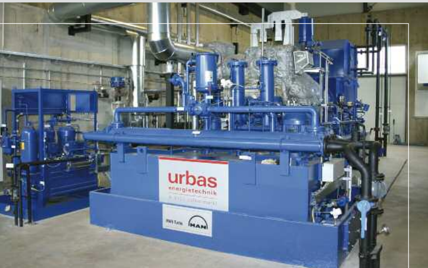
Bioenergy Bardejov s.r.o. location: Bardejov, Slovakia industrial: District heating output: 35 t/h, 65 bar 8 MW el 20 MW th
