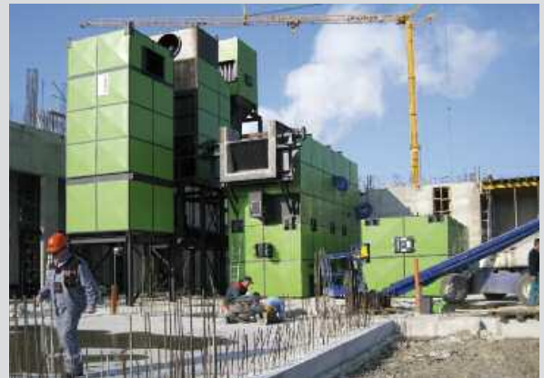
picture of installation
