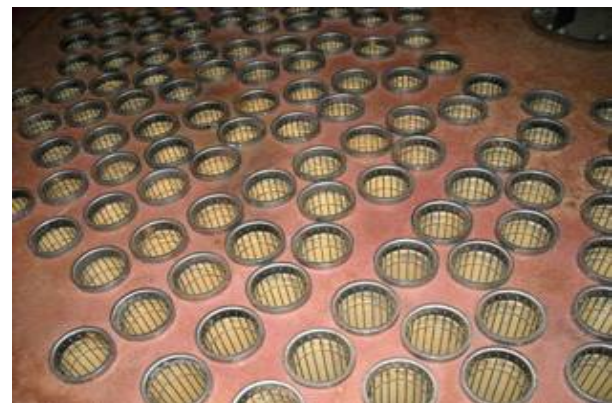
Clean air chamber filter unit after start-up operation
