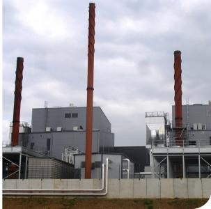
The latest delivery is a combined heat and power production plant to the municipality of Ham in the province of Limburg. The BioPower 9 modular biomass power plant utilizes bubbling fluidized bed (BFB) technology and uses clean biomass as the main fuel.
