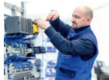
Final assembly, quality control
